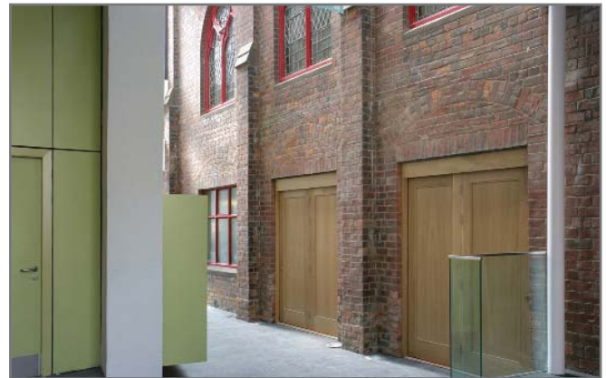
Daylight floods into the foyer and sanctuary windows between new & old.
